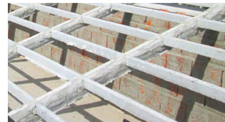
| Pre-stressed beam and rafter
